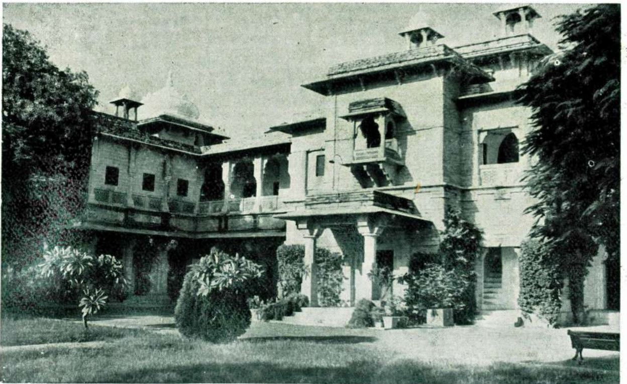
Ajmer Senior Boarding House — Constructed in 1882
