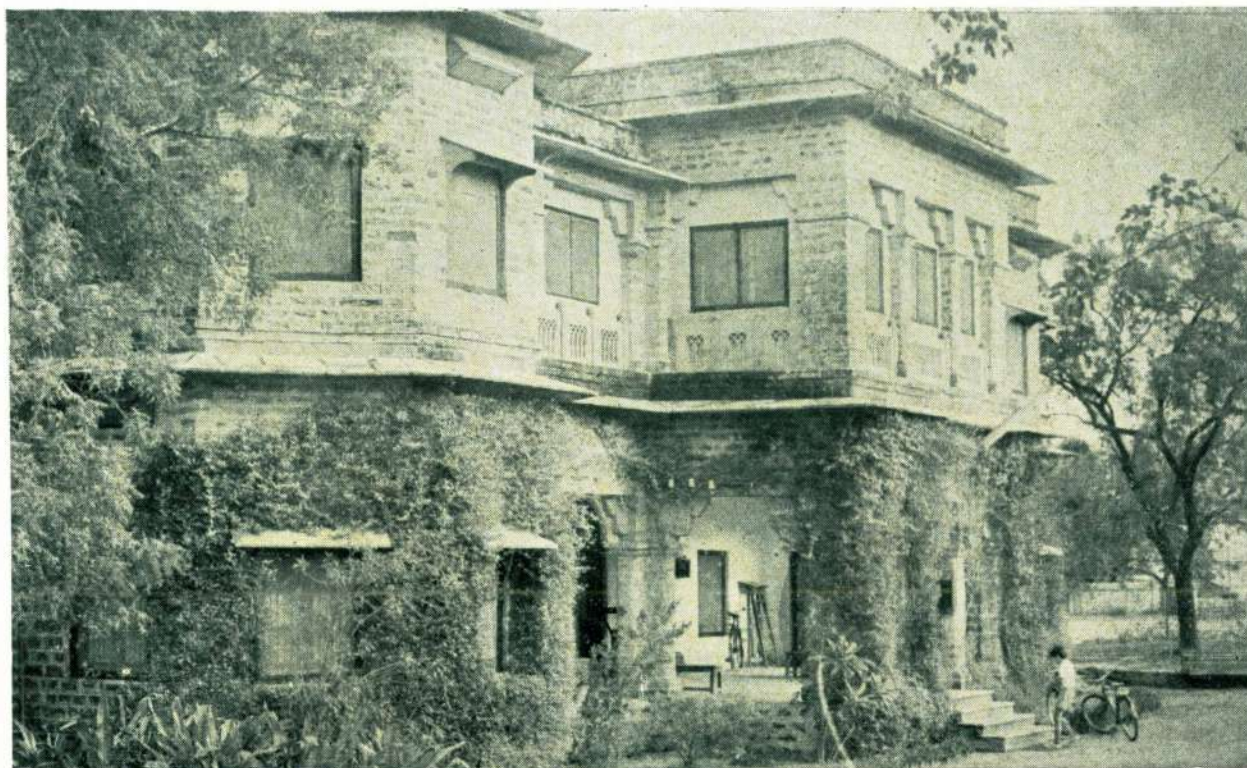
New Bharatpur Middle Boarding House — East Wing : Constructed in 1915
