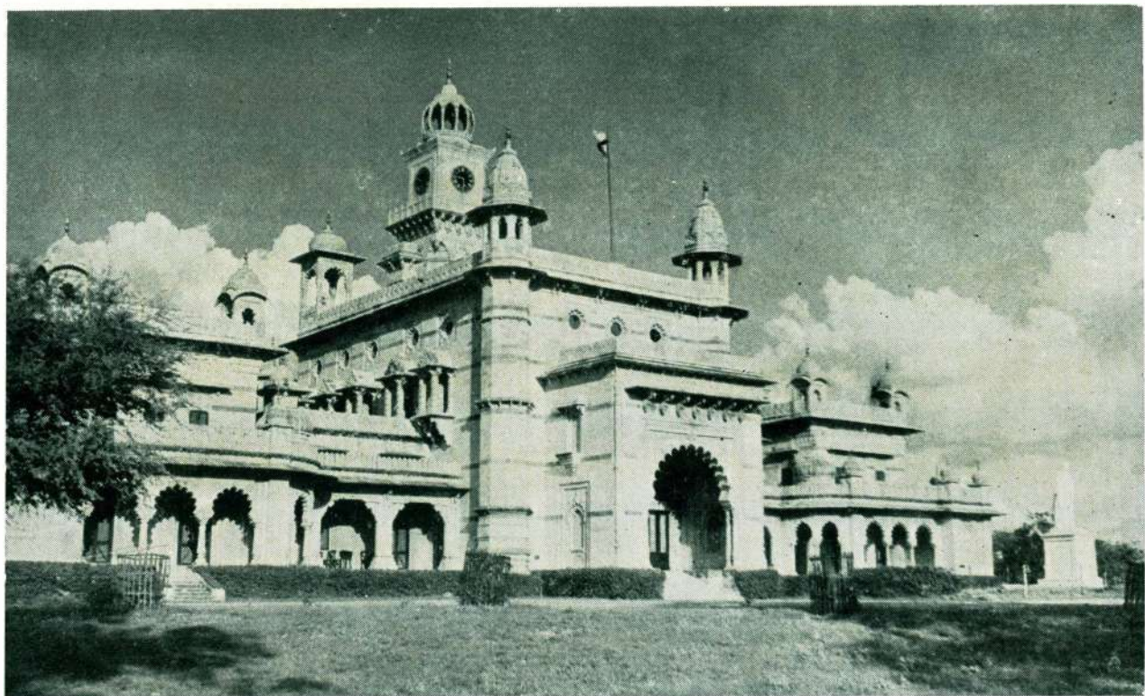
Main Building after completion
