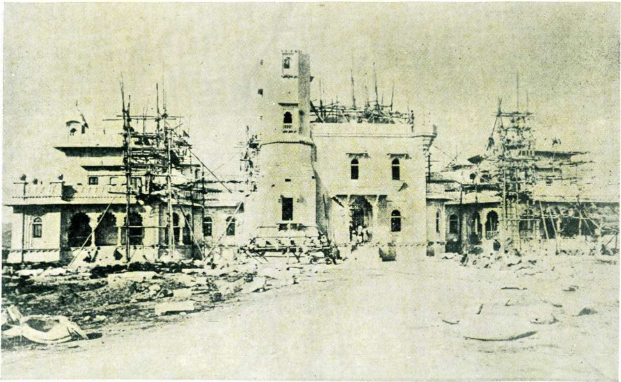
Main Building under construction — East View ( without the East Wing ) 1882
