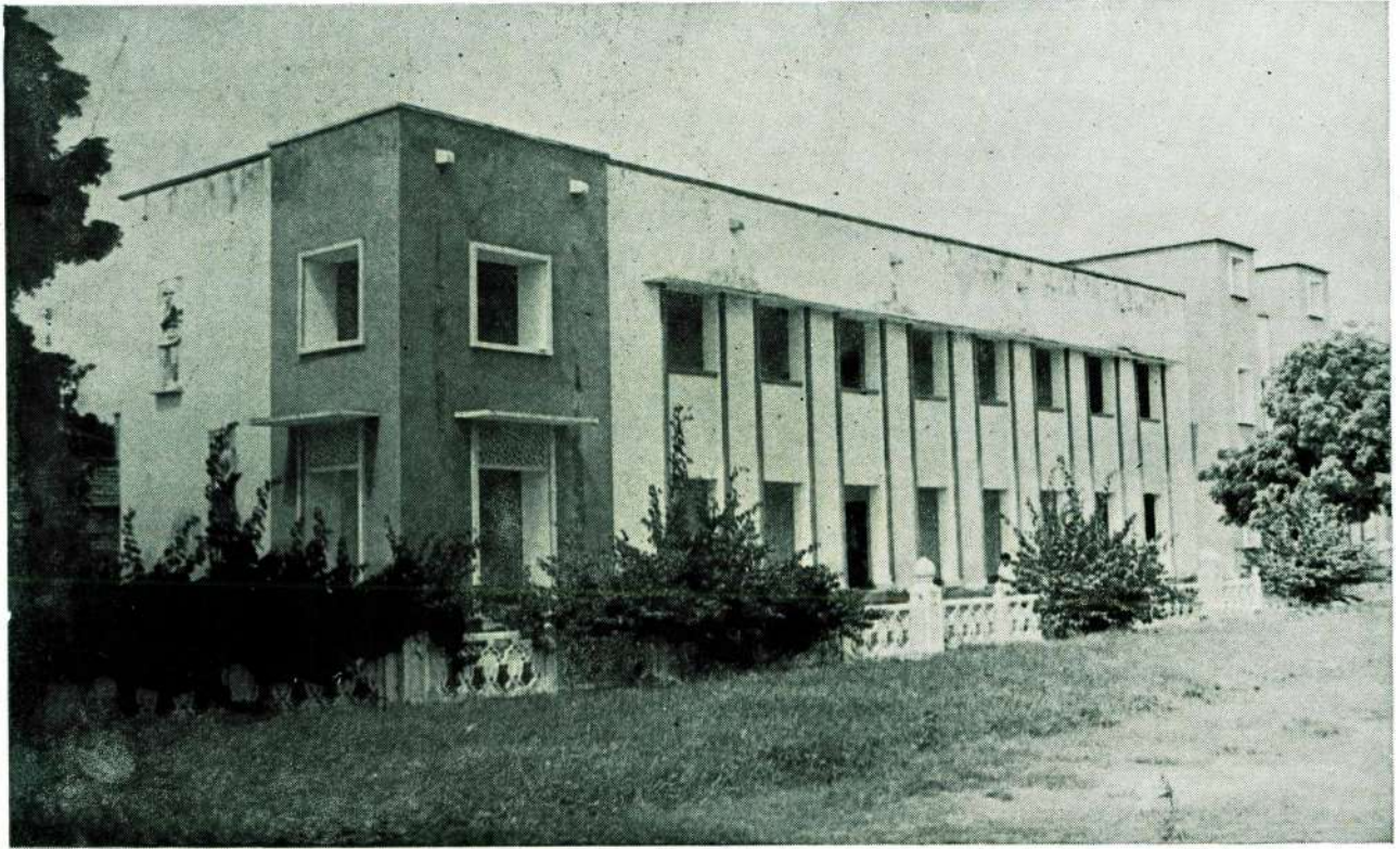
New Class Room Block : Constructed in 1960
